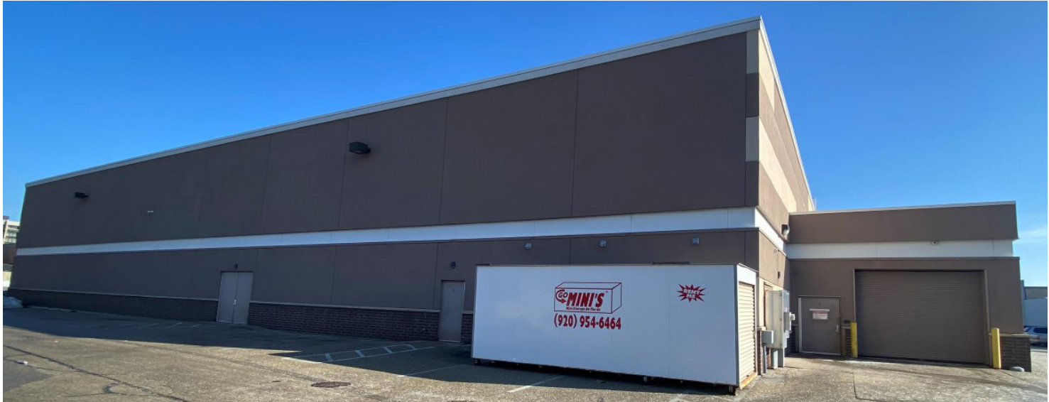
3 EXISTING EXTERIOR - WEST
