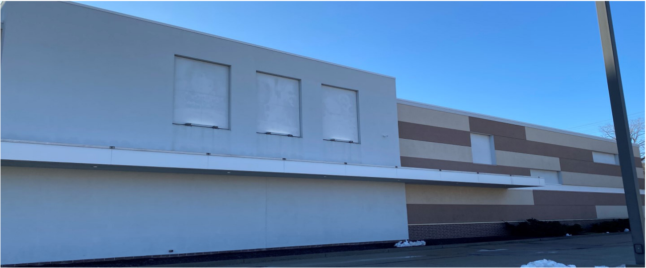
4 EXISTING EXTERIOR - NORTH
