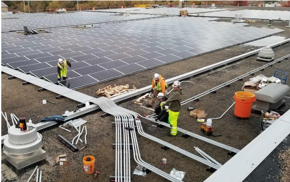
Photo: Department of Public Works Solar Array Installation
