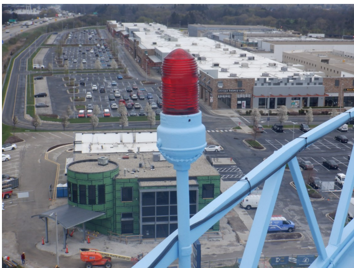
6) Aviation light (typical) on the balcony.
