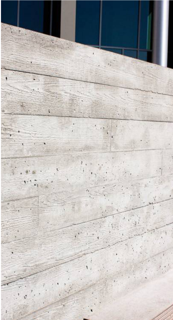
BFC-1 BOARD FORM CONCRETE
