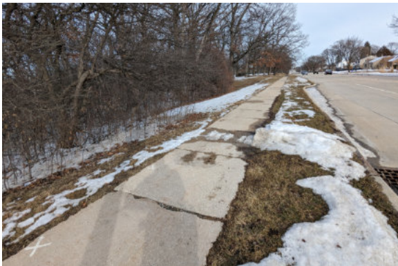
View east on Wisconsin Ave. Typical existing condition with 5' sidewalk and grass terrace. Terrace varies along corridor.
