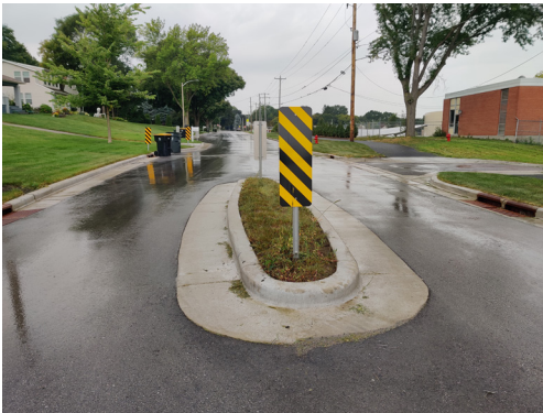
Chicanes were installed on Potter Road following a demonstration project in which barrels were installed on the street to create alternating curves to slow motorists
