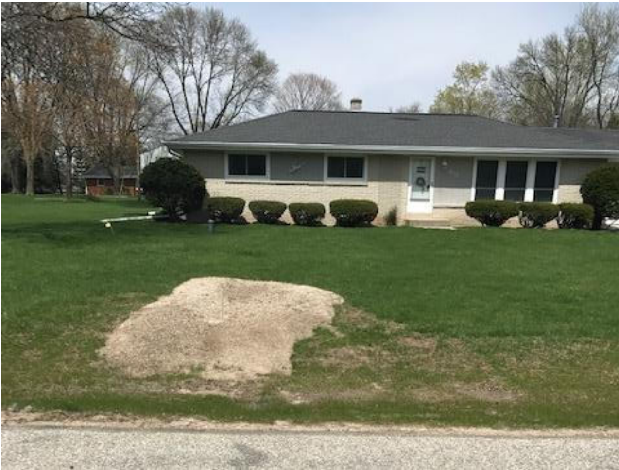
Above: Picture of backfill with ROUGH GRADE. In most cases this is how our contracts specify we will leave the job.
