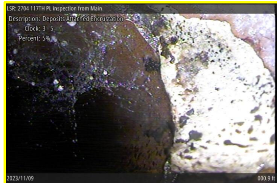
[Grade 2] Deposits Attached Encrustation at 000.9 ft, 3 - 5 o'clock
