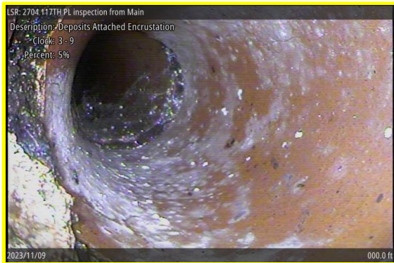
[Grade 2] Deposits Attached Encrustation at 000.0 ft, 3 - 9 o'clock
