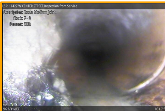
[Grade 3] Roots Medium Joint at 031.7 ft, 7 - 9 o'clock
