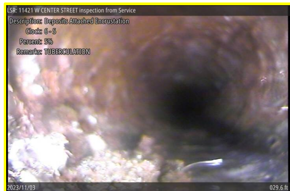
[Grade 2] Deposits Attached Encrustation at 029.6 ft, 6 - 5 o'clock | TUBERCULATION
