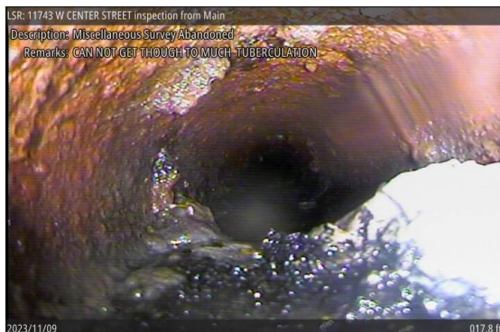
Miscellaneous Survey Abandoned at 017.8 ft | CAN NOT GET THROUGH TO MUCH TUBERCULATION
