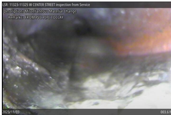
Miscellaneous Material Change at 003.6 ft | FROM PVC PIPE TO CLAY
