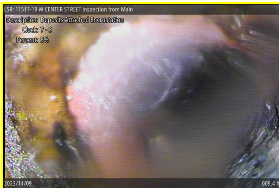
[Grade 2] Deposits Attached Encrustation at 009.4 ft, 7 - 5 o'clock
