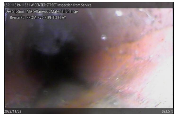
Miscellaneous Material Change at 022.5 ft | FROM PVC PIPE TO CLAY
