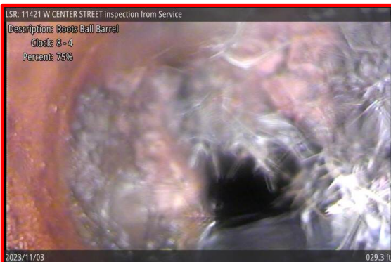
[Grade 5] Roots Ball Barrel at 029.3 ft, 8 - 4 o'clock
