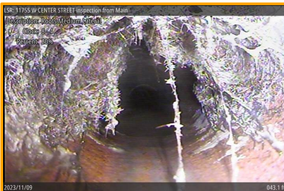
[Grade 3] Roots Medium Lateral at 043.1 ft, 8 - 4 o'clock
