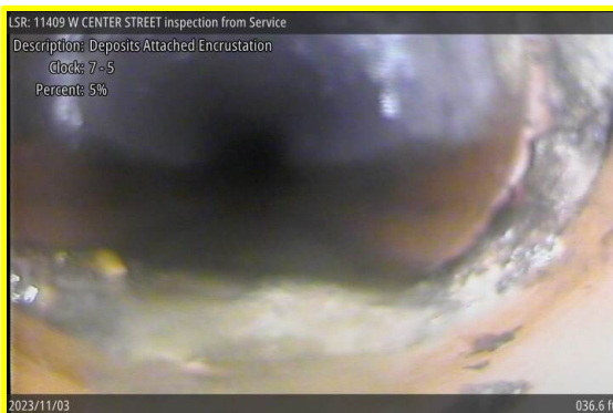
[Grade 2] Deposits Attached Encrustation at 036.6 ft, 7 - 5 o'clock
