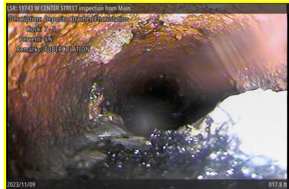
[Grade 2] Deposits Attached Encrustation at 017.8 ft, 7 - 5 o'clock | TUBERCULATION
