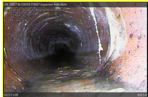
[Grade 2] Deposits Attached Encrustation at 020.5 ft, 7 - 5 o'clock
