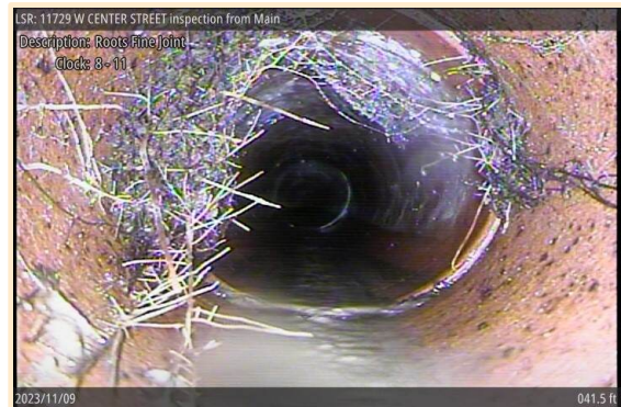
[Grade 1] Roots Fine Joint at 041.5 ft, 8 - 11 o'clock
