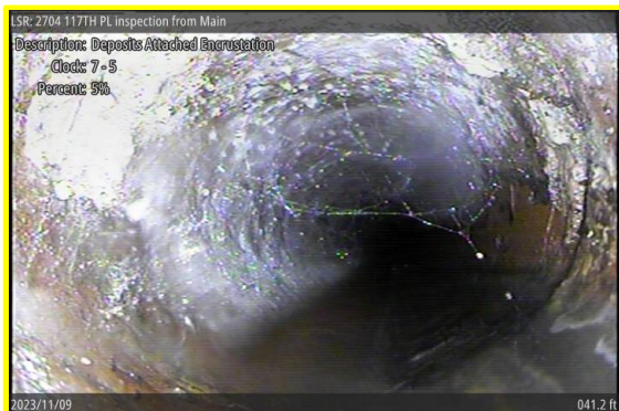
[Grade 2] Deposits Attached Encrustation at 041.2 ft, 7 - 5 o'clock
