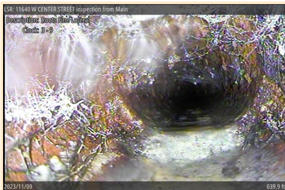
[Grade 1] Roots Fine Lateral at 039.9 ft, 3 - 9 o'clock
