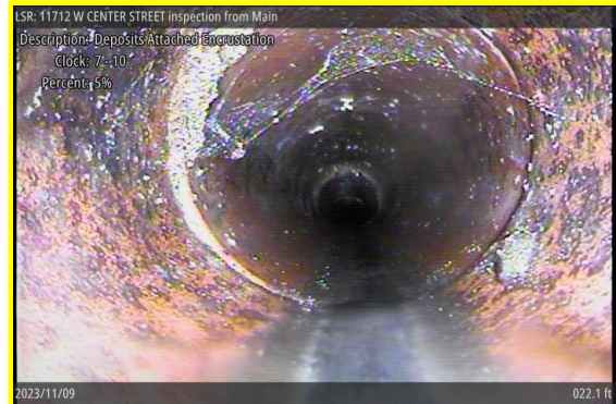
[Grade 2] Deposits Attached Encrustation at 022.1 ft, 7 - 10 o'clock
