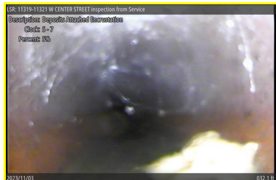
[Grade 2] Deposits Attached Encrustation at 032.1 ft, 5 - 7 o'clock
