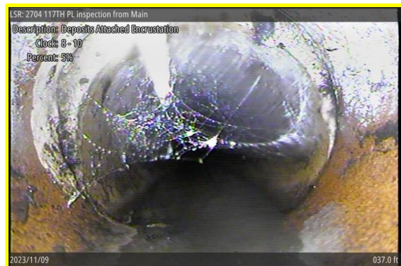
[Grade 2] Deposits Attached Encrustation at 037.0 ft, 8 - 10 o'clock
