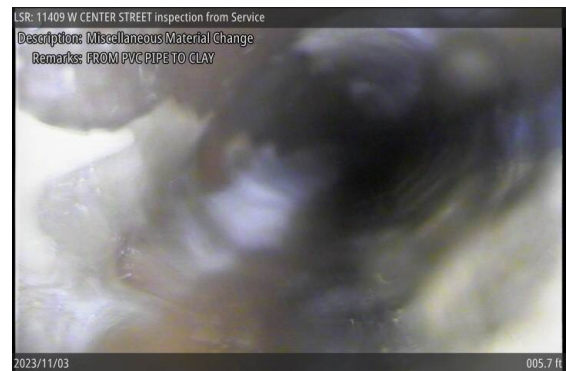
Miscellaneous Material Change at 005.7 ft | FROM PVC PIPE TO CLAY
