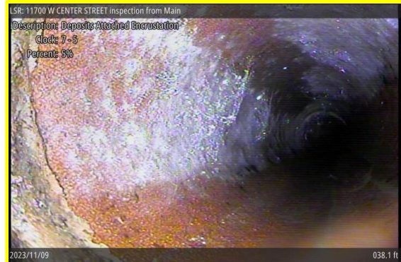
[Grade 2] Deposits Attached Encrustation at 038.1 ft, 7 - 5 o'clock
