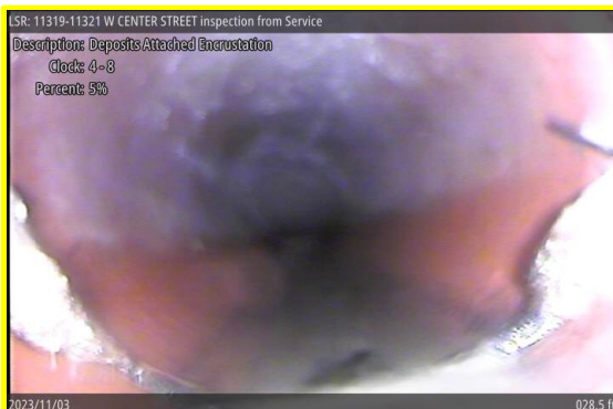
[Grade 2] Deposits Attached Encrustation at 028.5 ft, 4 - 8 o'clock
