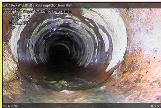
[Grade 2] Deposits Attached Encrustation at 032.5 ft, 7 - 5 o'clock
