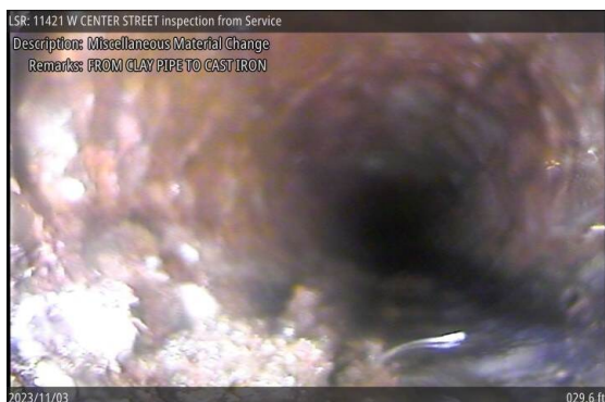
Miscellaneous Material Change at 029.6 ft | FROM CLAY PIPE TO CAST IRON
