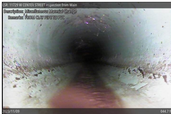
Miscellaneous Material Change at 044.7 ft | FROM CLAY PIPE TO PVC
