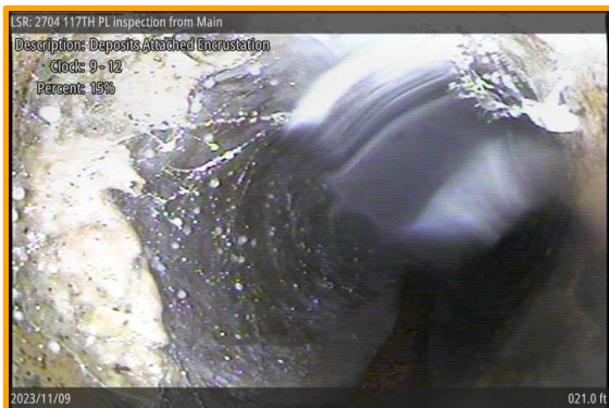
[Grade 3] Deposits Attached Encrustation at 021.0 ft, 9 - 12 o'clock
