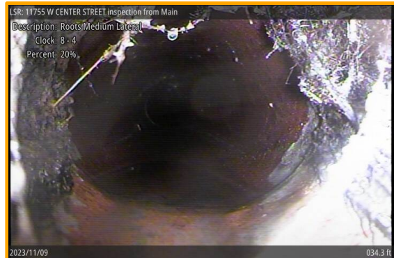
[Grade 3] Roots Medium Lateral at 034.3 ft, 8 - 4 o'clock
