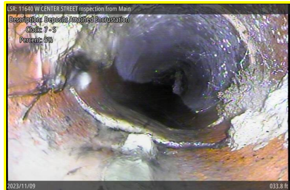
[Grade 2] Deposits Attached Encrustation at 033.8 ft, 7 - 5 o'clock
