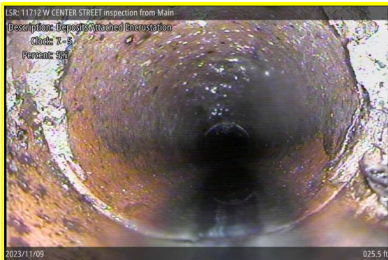
[Grade 2] Deposits Attached Encrustation at 025.5 ft, 7 - 5 o'clock
