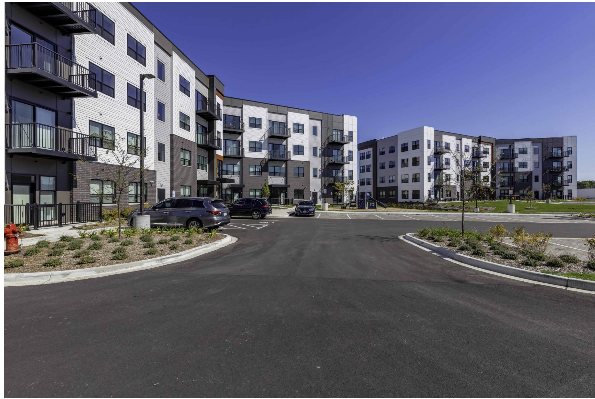
VIEW LOOKING FROM WEST TOWARDS BUILDING
