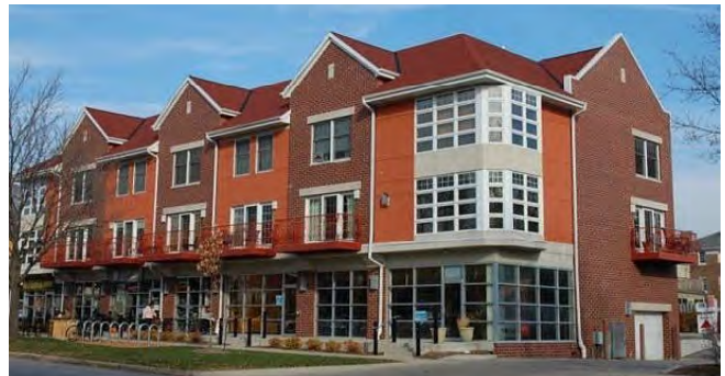
Mixed-Use Development 9125 W North Avenue Wauwatosa, WI
