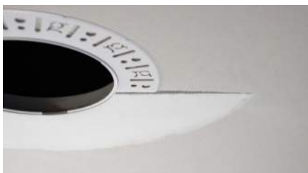
Partially finished mud ring, showing cross-section detail.
