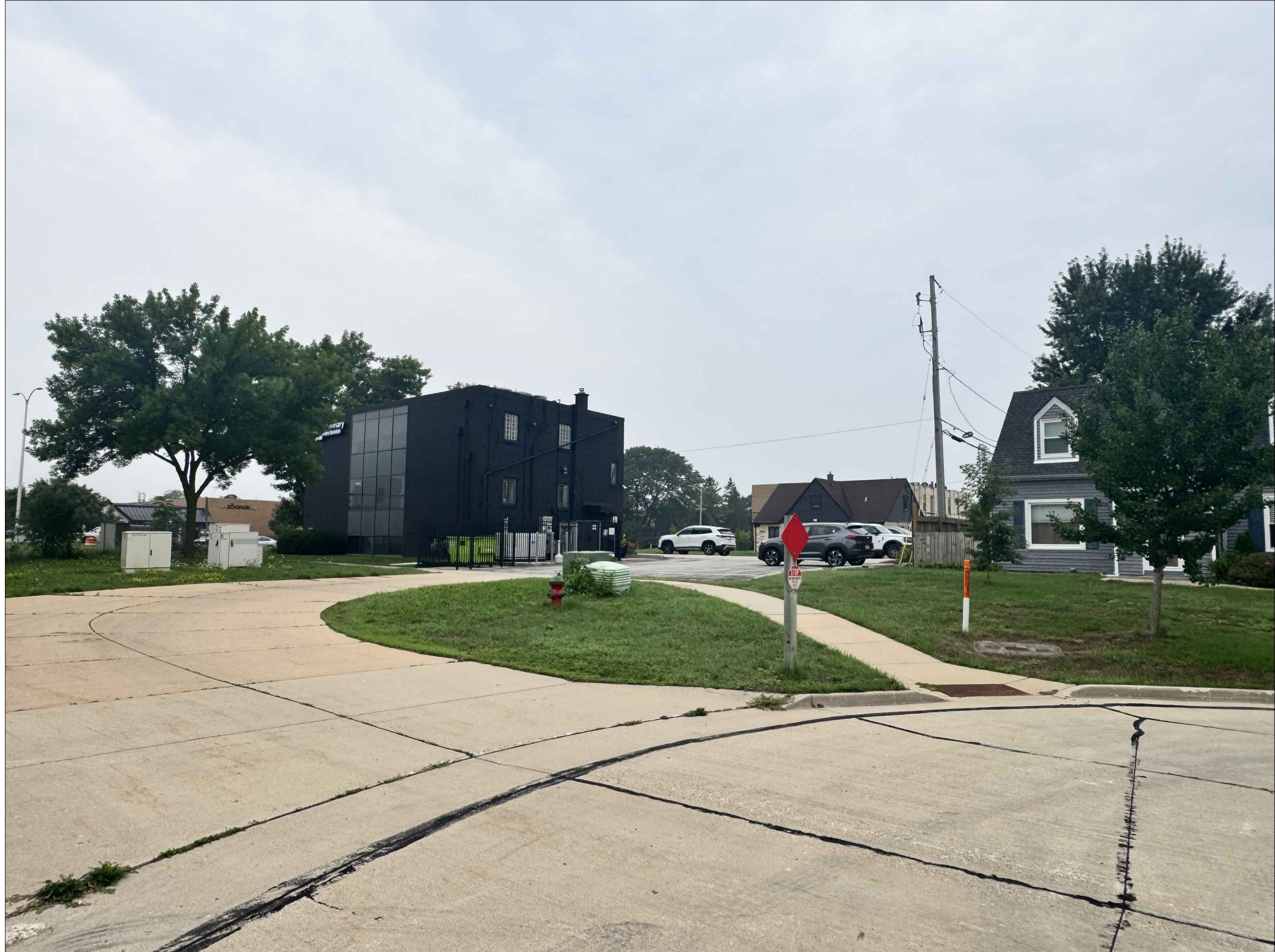
Rear Elevation from NE
