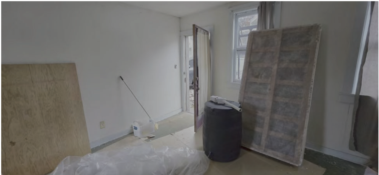
View of Existing Entry Door
