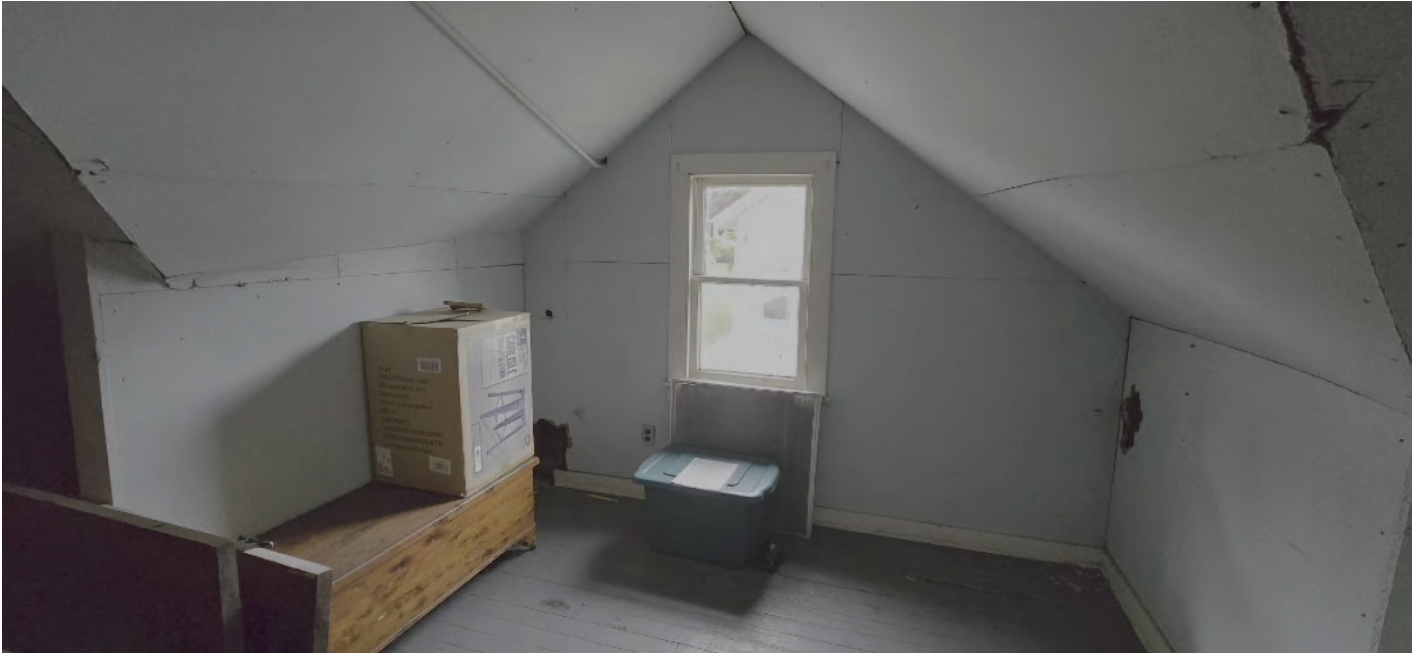
View of Existing Second Floor
