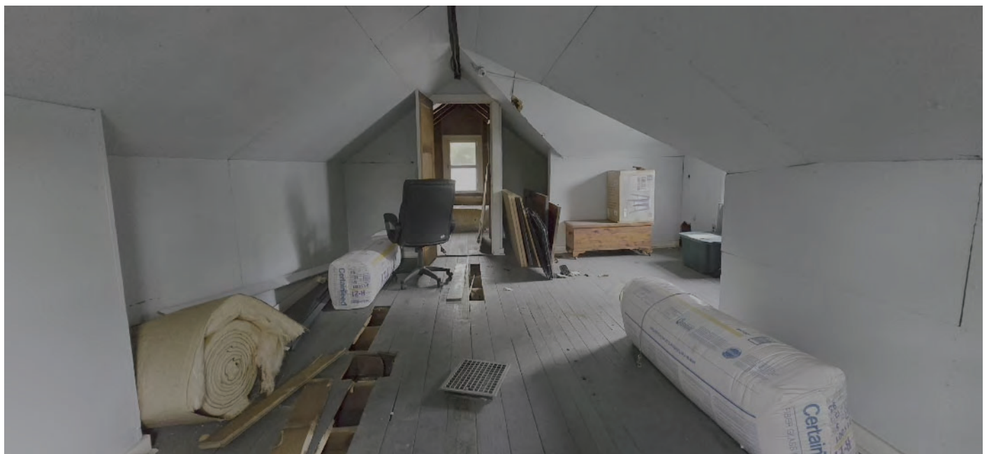
View of Existing Second Floor
