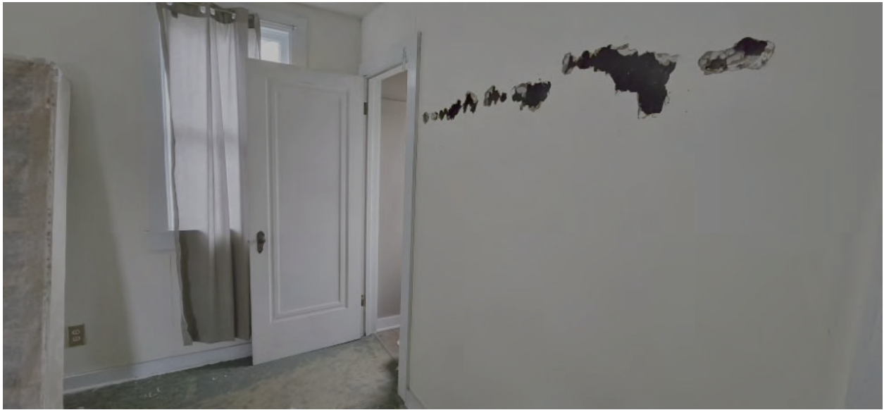
View of Existing Stair Wall
