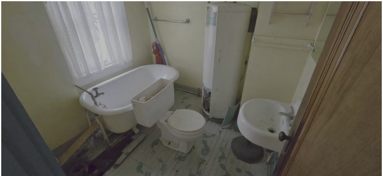
View of Existing Bathroom
