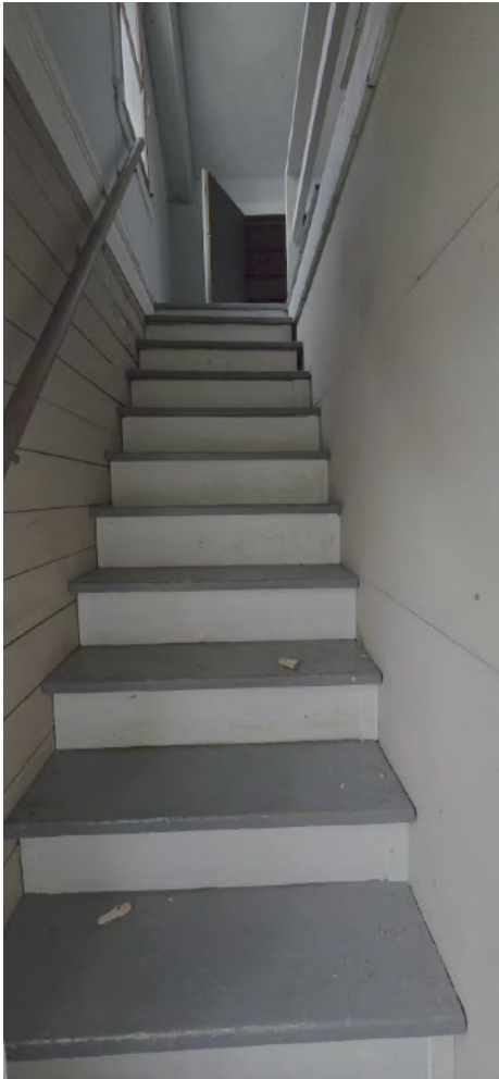
View of Existing Stair
