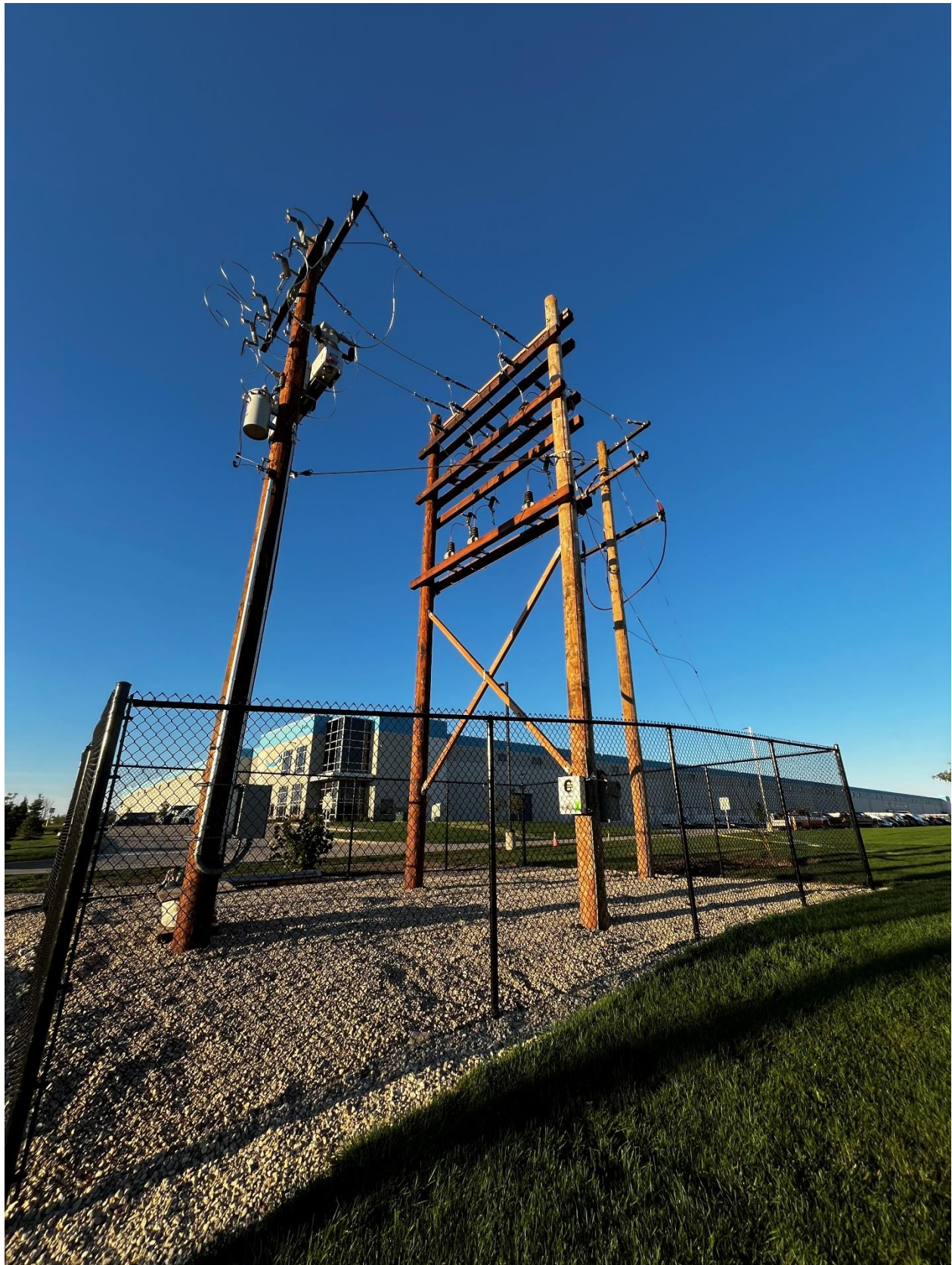
Figure 2: Image of an identical substation and 7-foot-tall black vinyl coated chain link fence installed around a new substation at another Amazon location in Wisconsin
