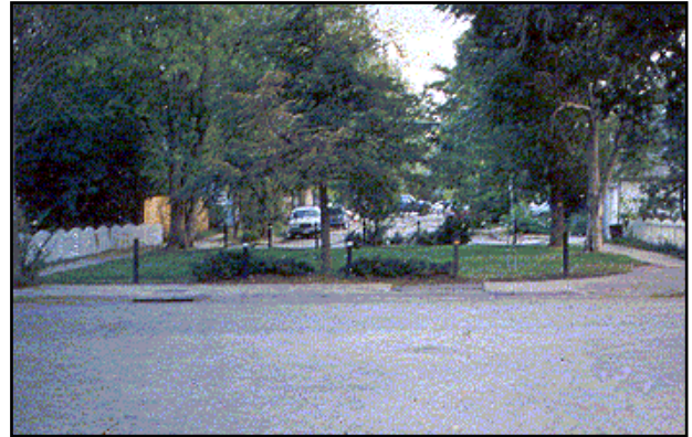
Street closure used as a traffic calming measure Resource: ITE Traffic Calming
