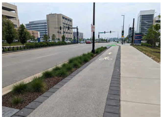
Protected Bike Lane
