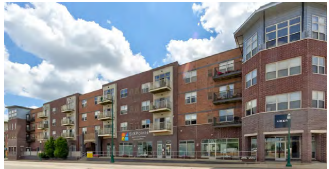
Six Point Apartment Homes 6519 W. Greenfield Avenue West Allis, WI
