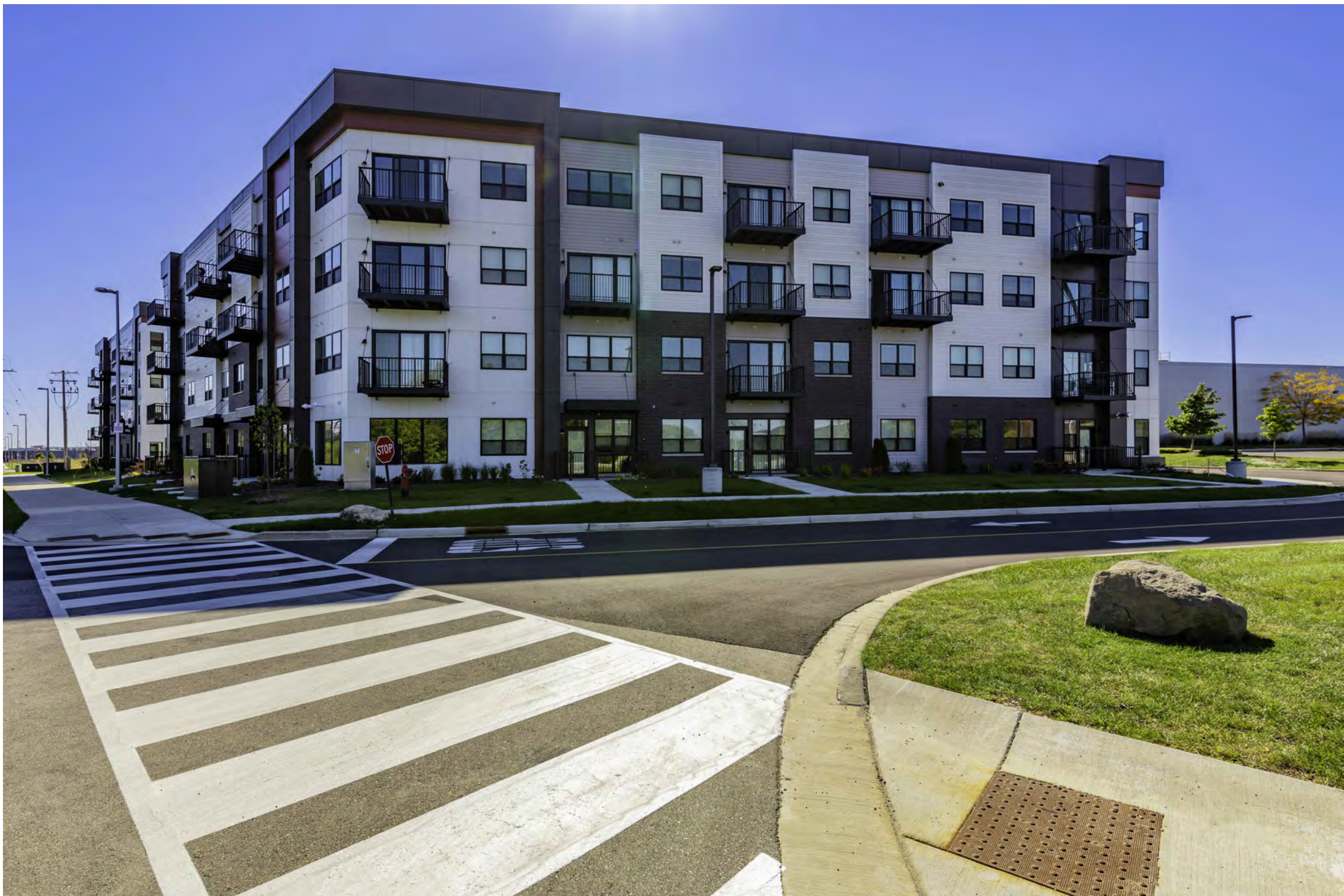
VIEW LOOKING FROM SITE TO EXISTING BUILDING
