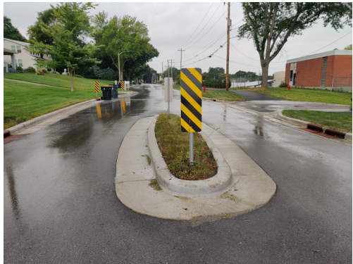
Chicanes were installed on Potter Road following a demonstration project in which barrels were installed on the street to create alternating curves to slow motorists
