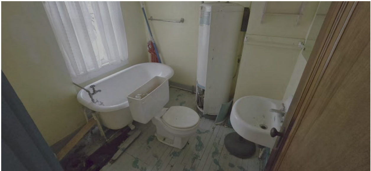
View of Existing Bathroom
