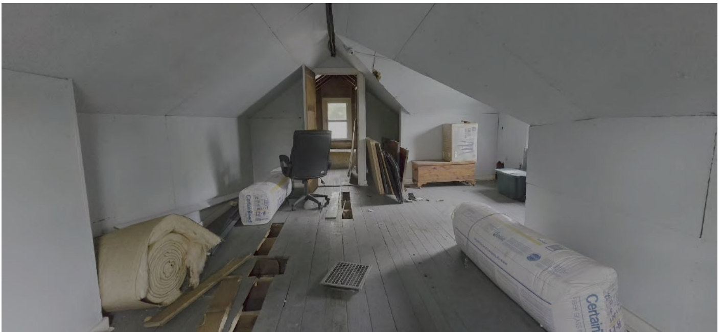
View of Existing Second Floor
