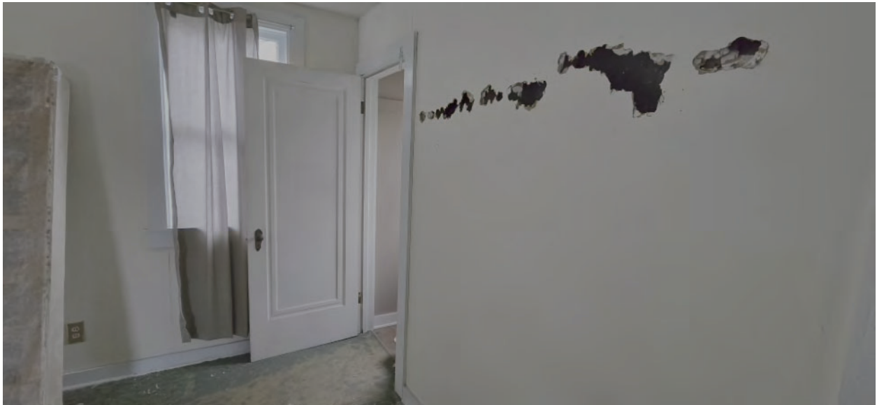
View of Existing Stair Wall
