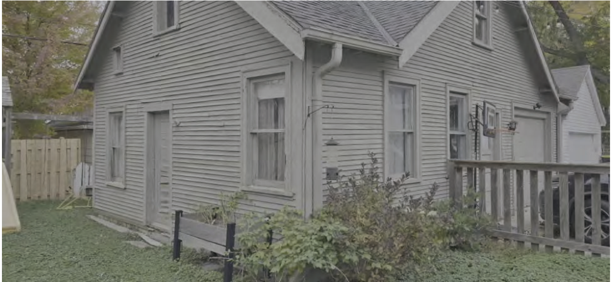
South and East Facing Elevation
