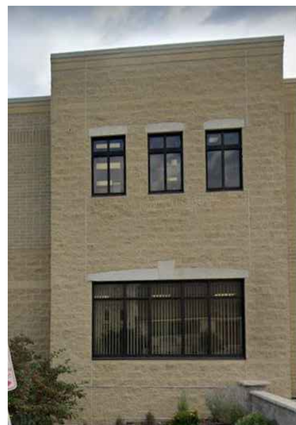
SPLITFACE AND SMOOTH FACE CMU; PRECAST STONE HEADERS AND SILLS
