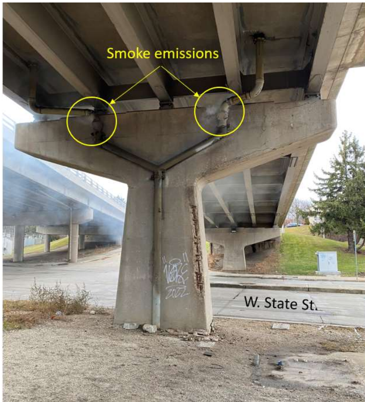
Figure 2-4 Smoke Emissions from Box Culvert Connection UNK-2-B-4-6 (aka 152019)
