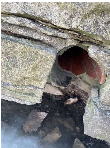
Figure 2-1. Existing VCP Penetration of WPA Wall
