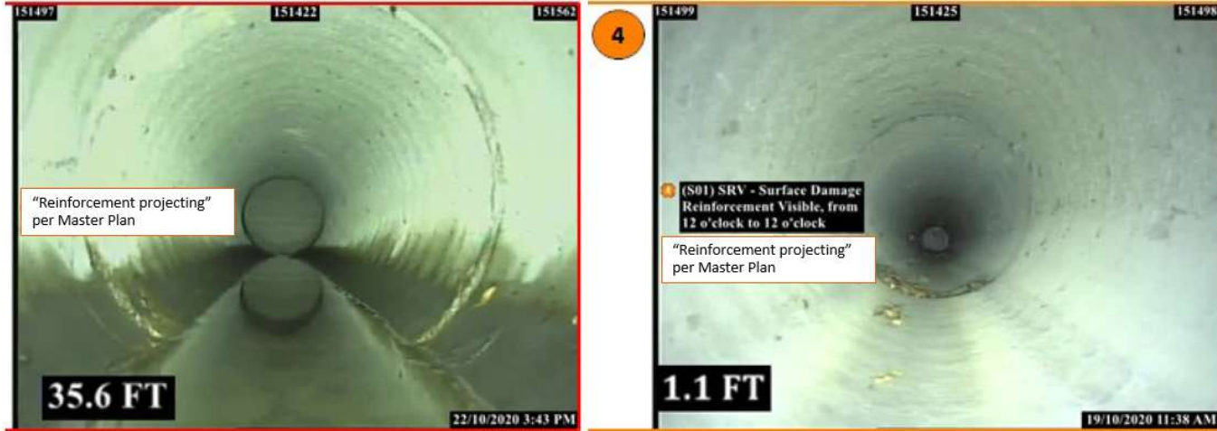
Figure 2-7 Examples of Reinforcement Projecting from Master Plan
