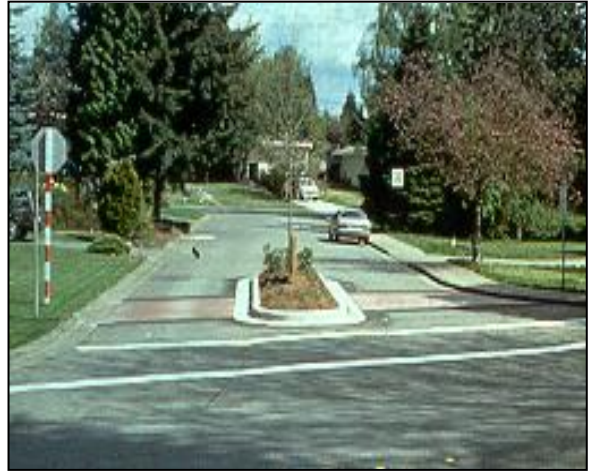
Center Island Narrowing, also called a Gateway Resource: ITE Toolbox of Traffic Calming Measures
