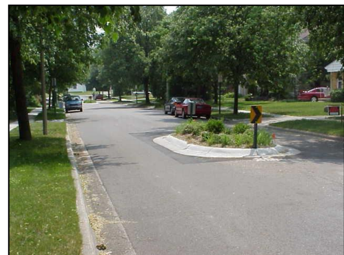
Example of chicane Resource: ITE Procedures and Warrants
