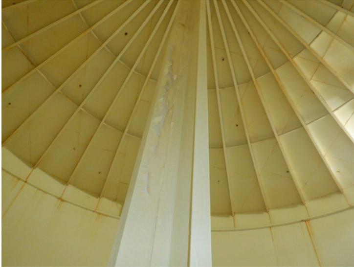
37) There are no significant coating failures on the center column.
