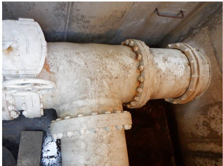
47) The pit piping coating is in good condition with minor corrosion.
