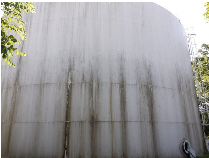
9) There is heavy mildew on the sidewall but no significant coating deterioration.
