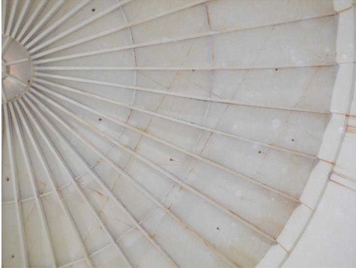
28) There are coating failures on the wet interior roof at the lap seams and roof stiffeners.
