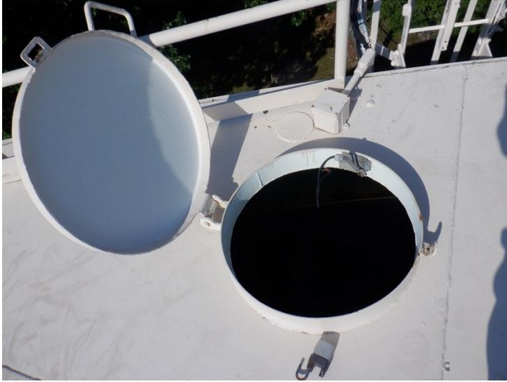
16) There was no gasket on the wet interior roof hatch.
