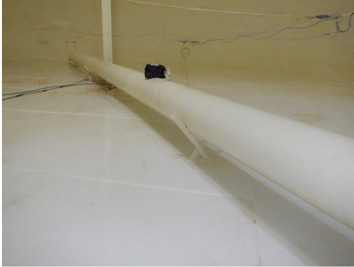
43) The fill pipe routes across the floor and discharges near the opposite sidewall.
