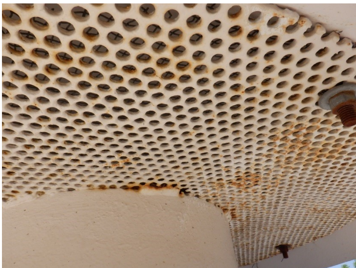
24) The roof vent screen is in good condition but oversized.
