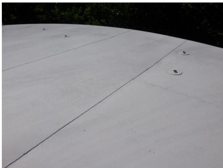
18) The roof coating is in good condition overall with no significant failures.
