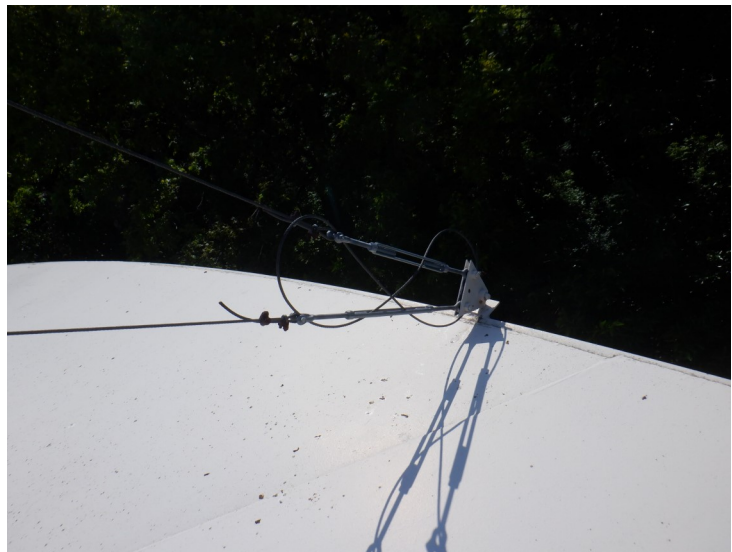
26) The attachment points for the three guyed wires at the edge of the roof for the antenna structure appear to be in good condition.
