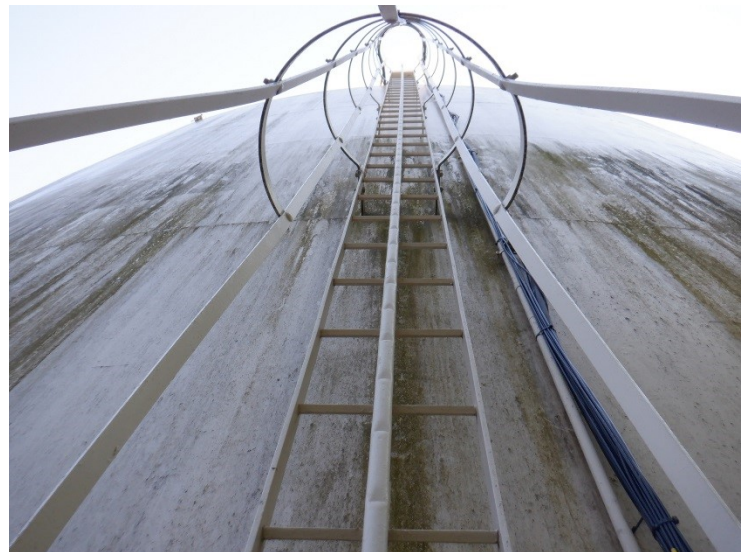
14) The sidewall ladder is in good condition. The ladder is equipped with a cage and a fall prevention device.
