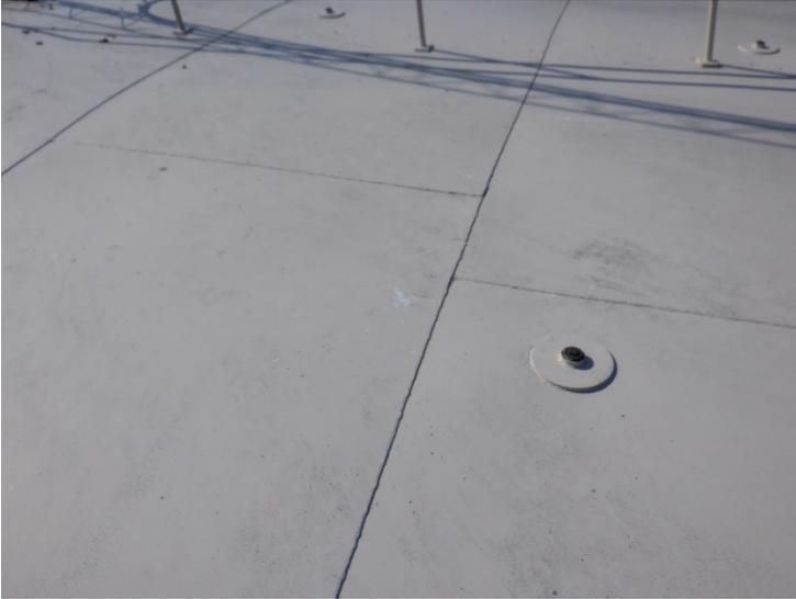
22) The roof rigging couplings are properly plugged.
