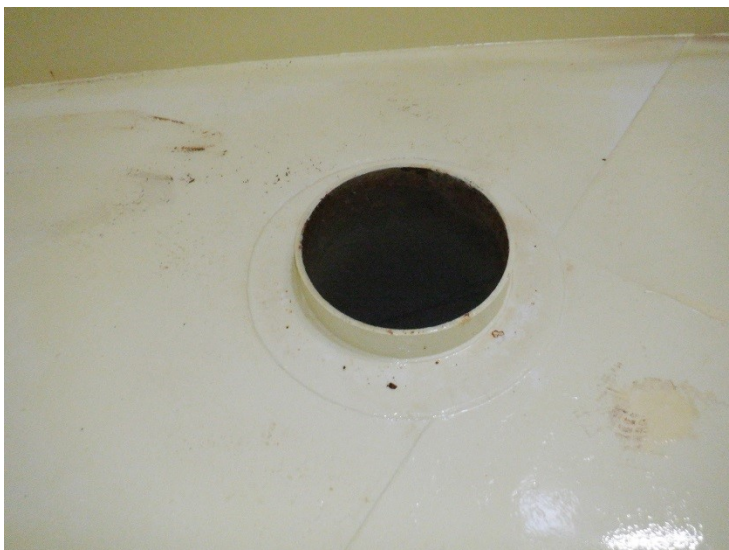
45) There are no deflector bars over the draw pipe in the wet interior.
