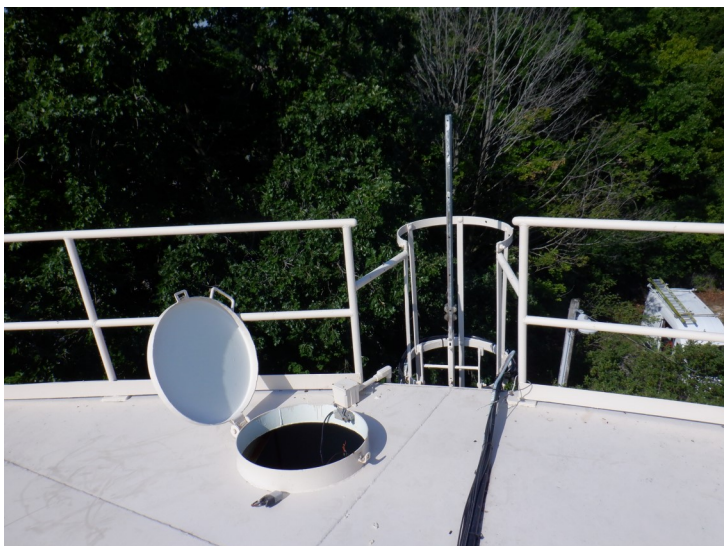
15) There are handrails on the roof on each side of the sidewall ladder. There is not a swing gate at the opening in the railing.
