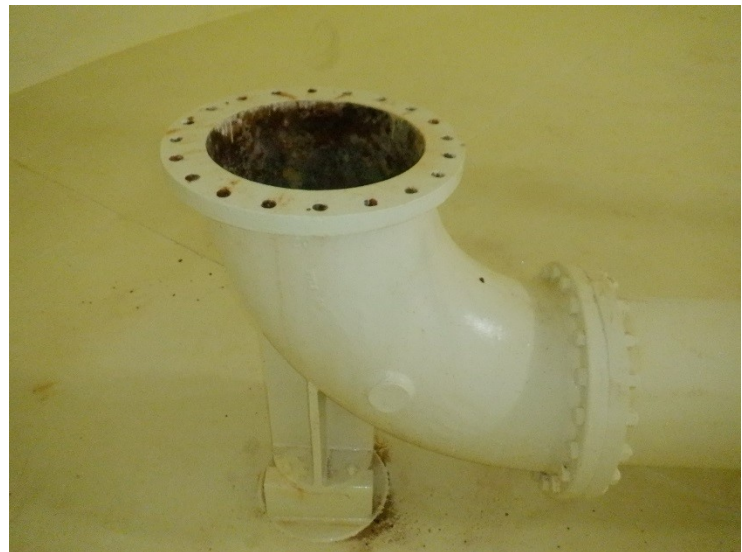
44) The fill pipe discharge is in good condition.
