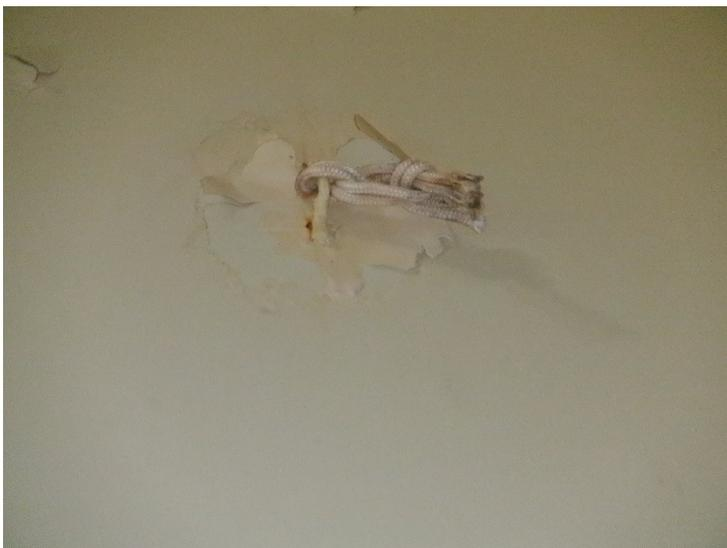
42) One rope for the cathodic protection system is broken.
