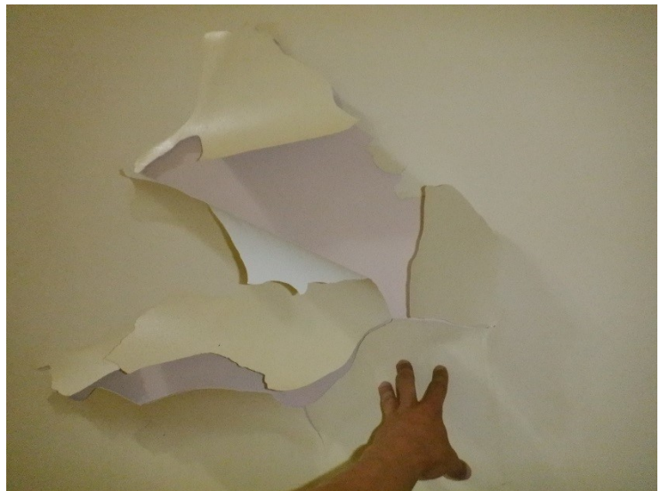
32) There is some topcoat delamination on the wet interior sidewall.
