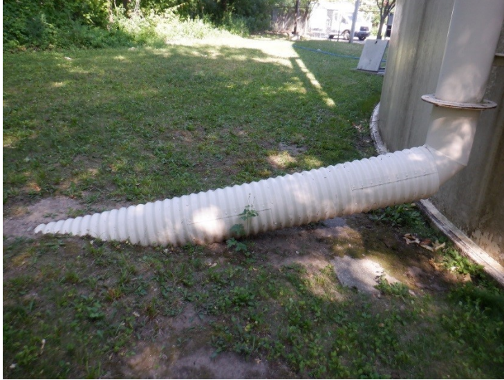
7) The overflow pipe exits the upper sidewall and routes below grade.
