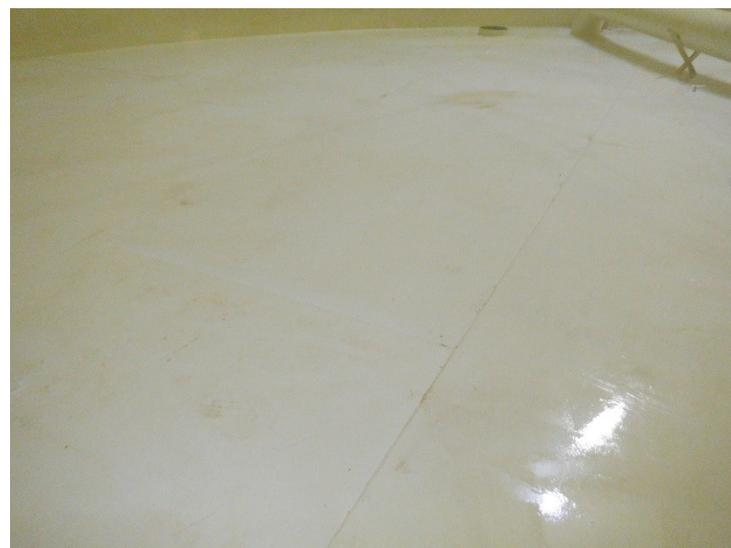
39) The coating on the floor is in good condition with no failures.
