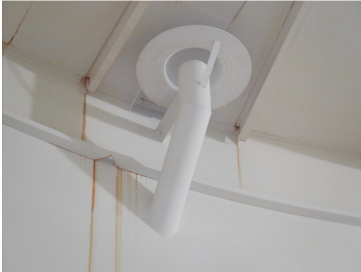
31) The overflow elbow and upper sidewall stiffener are in good condition.
