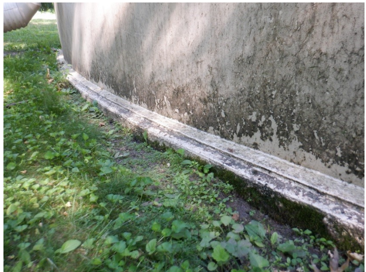
2) The concrete foundation is in good condition with no significant deterioration.
