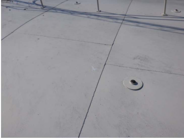
22) The roof rigging couplings are properly plugged.
