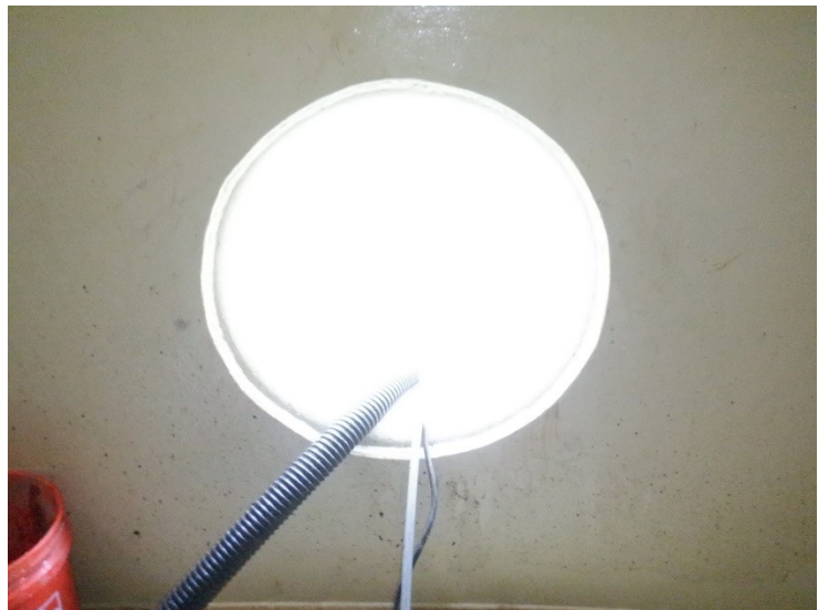
35) The two sidewall manways are in good condition.
