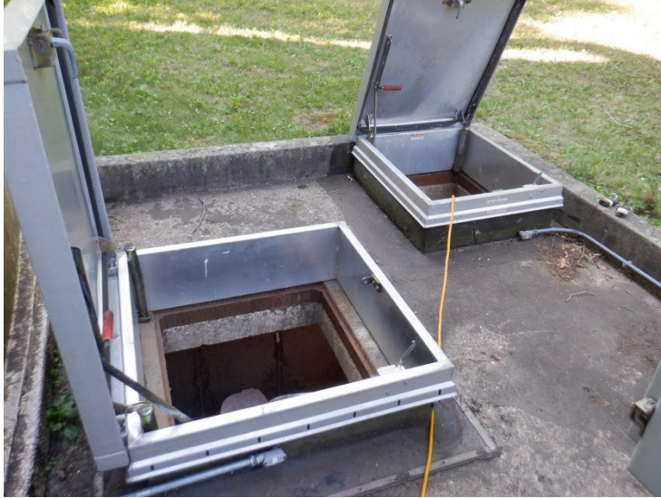
46) The metal hatches over the pit are in good condition.
