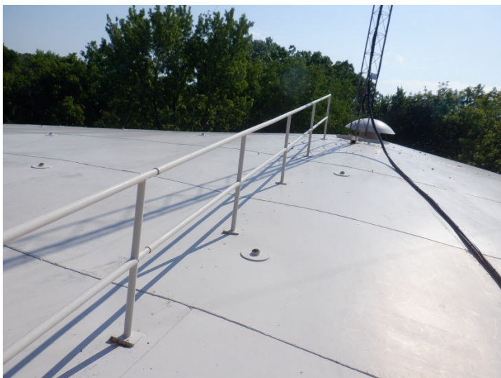
21) The handrail to the center of the tank is in good condition.
