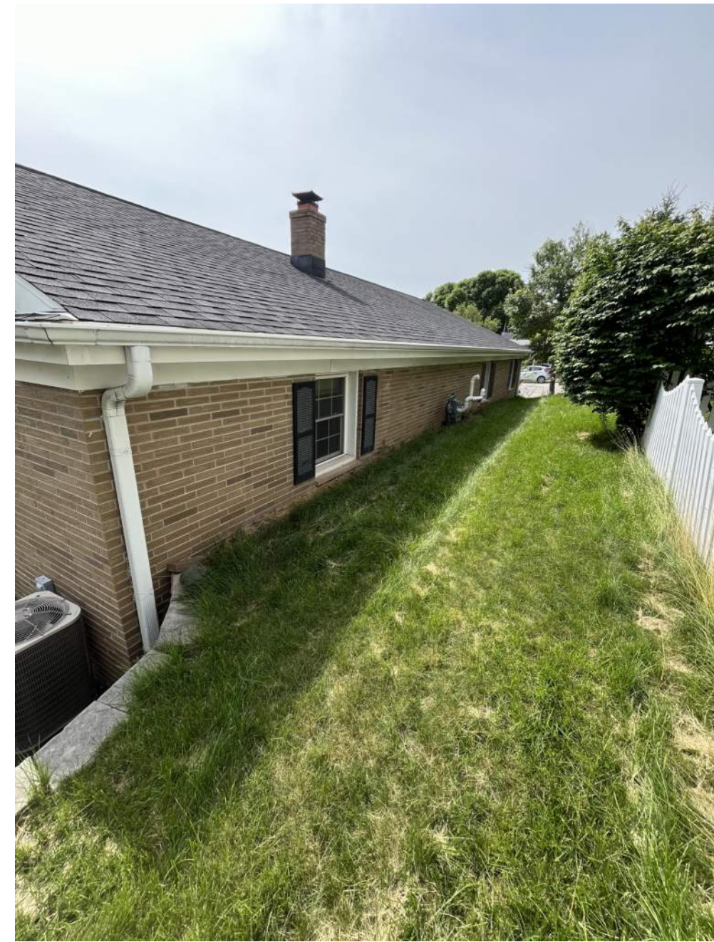
VIEW FROM REAR OF BUILDING
