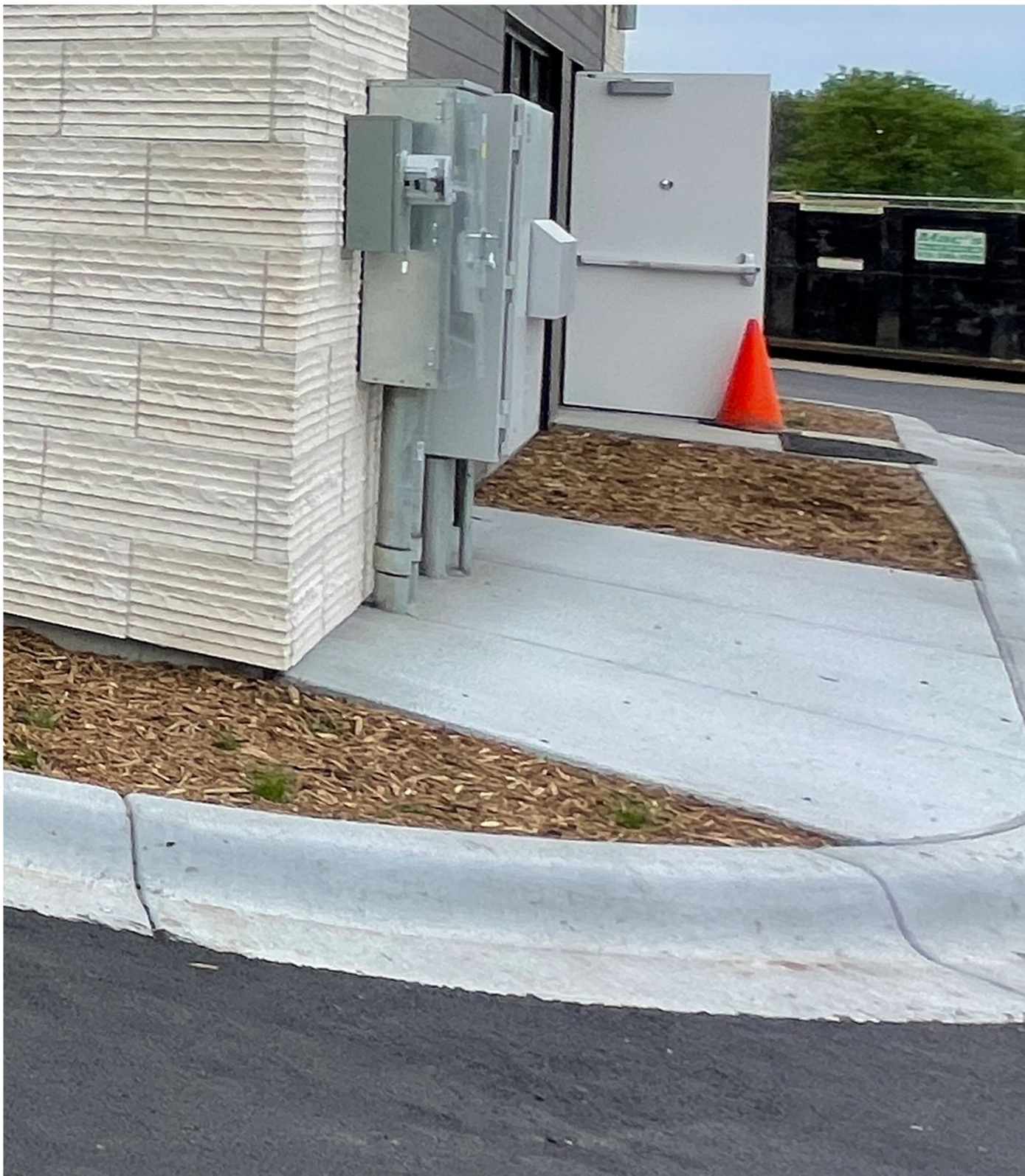
CAST STONE AT GRADE AND SIDEWALK
