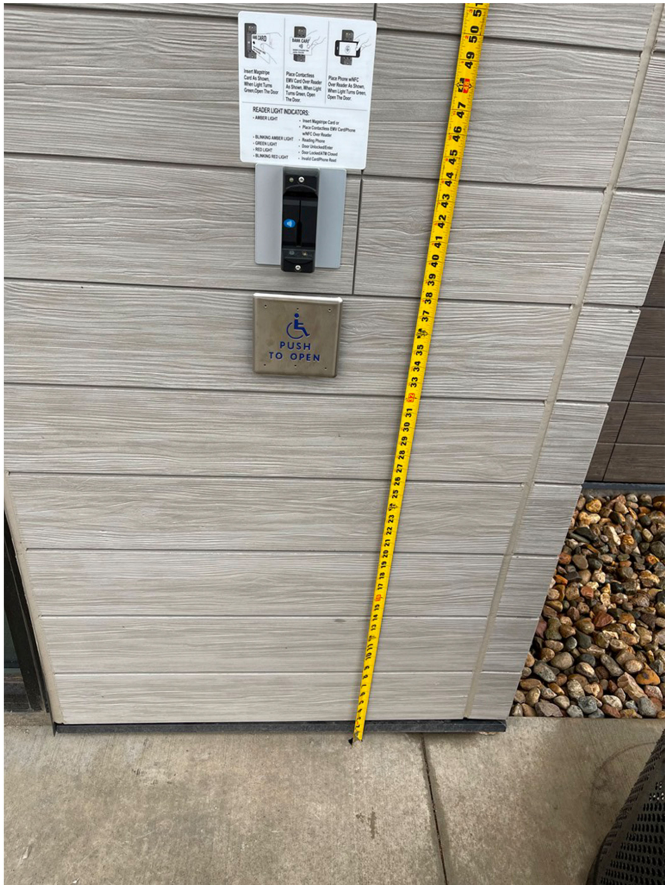
ENTRY FIBER CEMENT AT SIDEWALK
