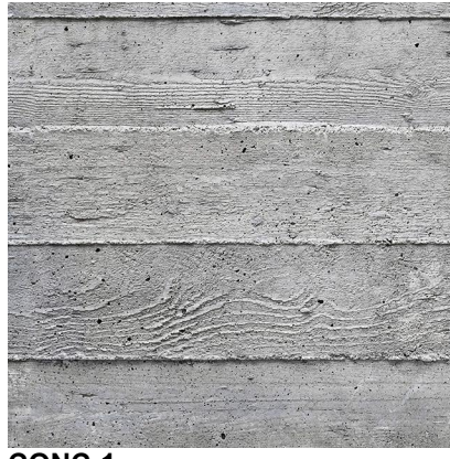
CONC-1 BOARD FORM CONCRETE
