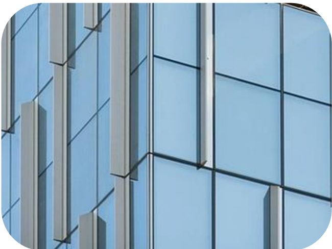
CURTAIN WALL MULLION & CAP EXTENSION TO MATCH WHITE METAL PANEL
