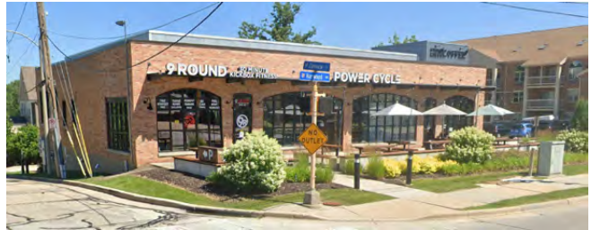
Adaptive reuse featuring facade and landscaping improvements, new signage, and expanded outdoor programming 7954 Harwood Avenue, Wauwatosa (2024)
