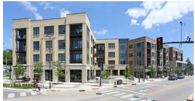
State Street Station 7400 W State Street Wauwatosa, WI
