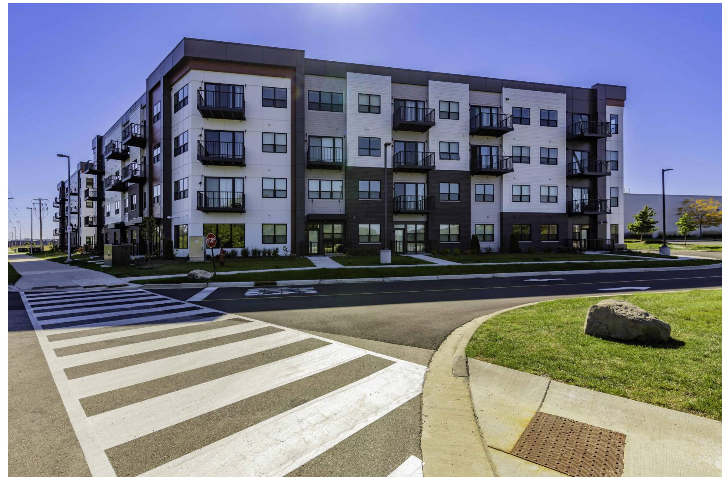
VIEW LOOKING FROM SITE TO EXISTING BUILDING
