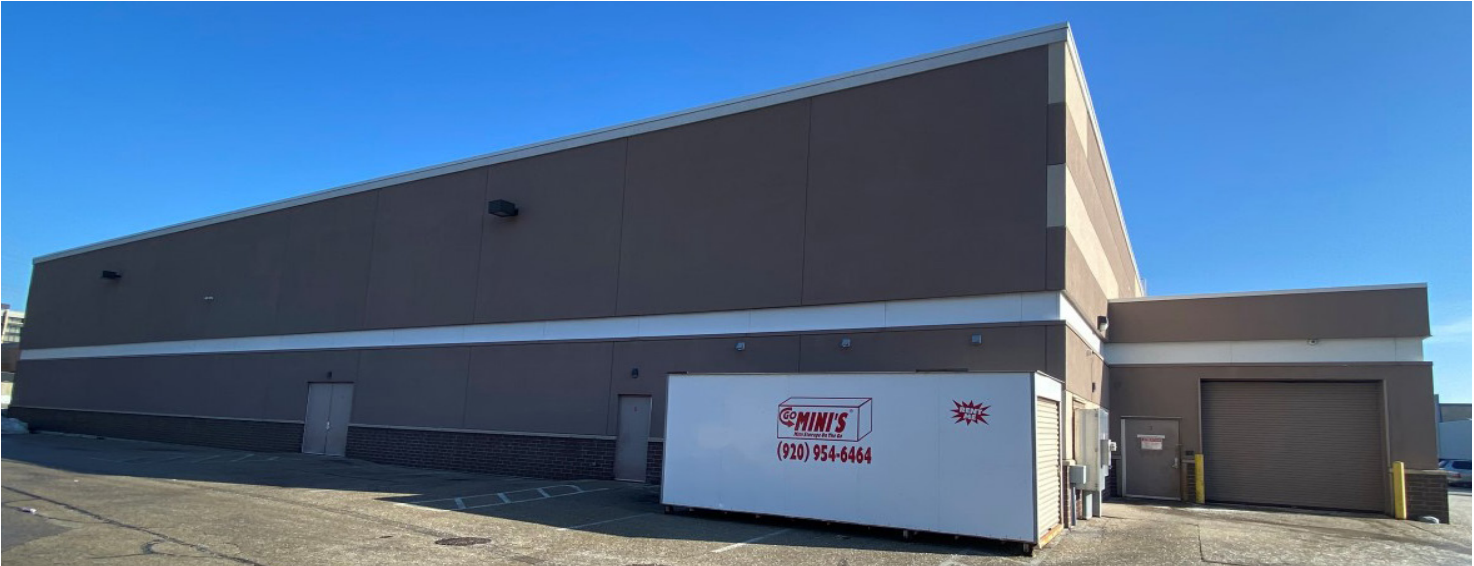
3 EXISTING EXTERIOR - WEST
